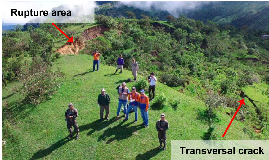
Illustration 3: Permanent landslide (rotational landslide) on Guarin Hill, Honduras. Source: El País.
