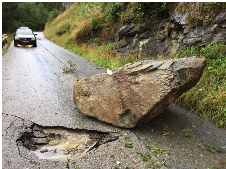
Illustration 15: Hole in the pavement left by a block upon impacting this road.
