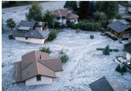
Illustration 14 **High intensity:** Reinforced concrete buildings can be destroyed by the high flow energy and large amounts of deposits. Source: Geotest AG.
