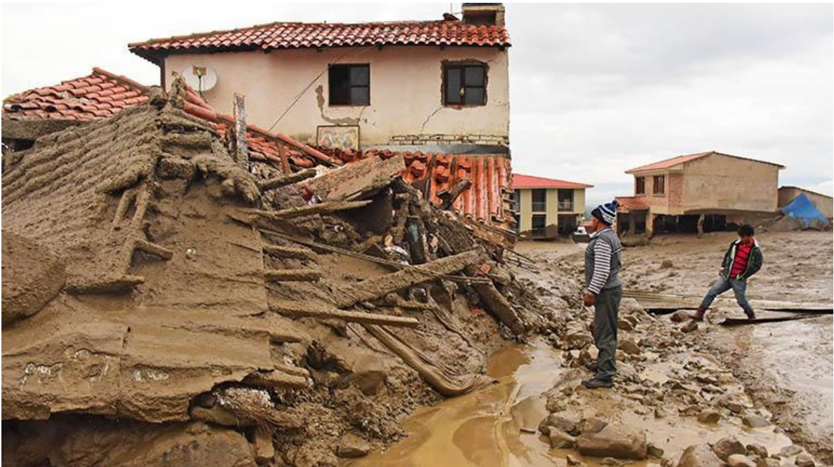
Illustration 1: Buildings destroyed and damaged Tiquipaya, Bolivia. Source: Los Tiempos.
